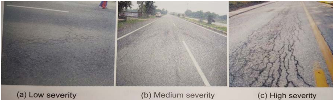
Photo 6.3.3 Alligator Cracks
