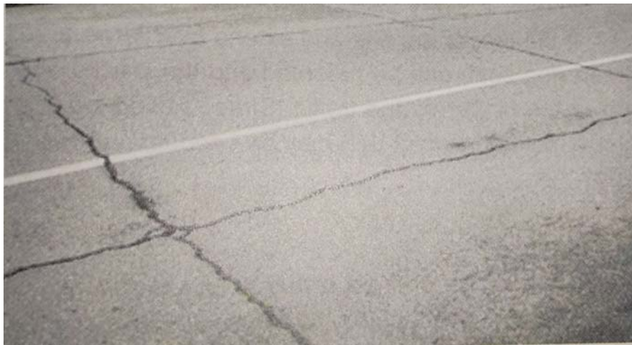
Photo 6.3.7 Reflection Cracking
